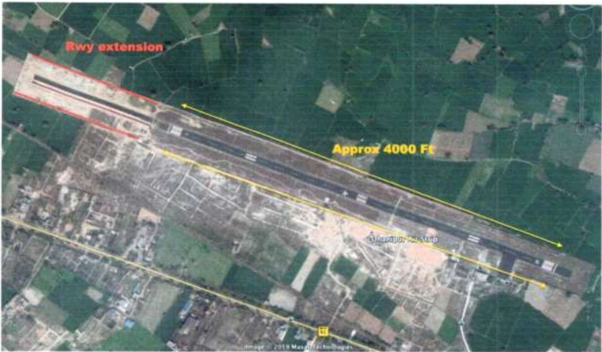
Fig-10: Extension Work of Runway
