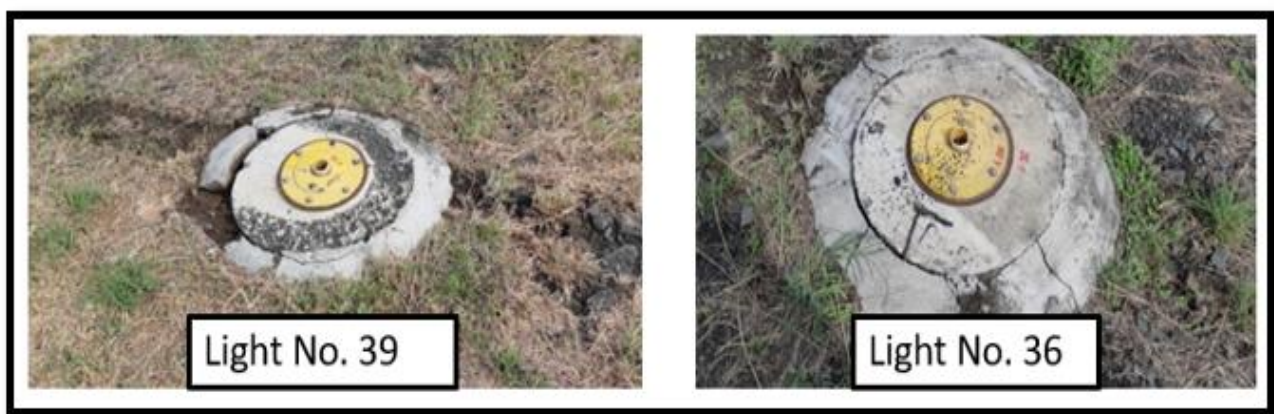
Fig 8: Broken runway edge lights
