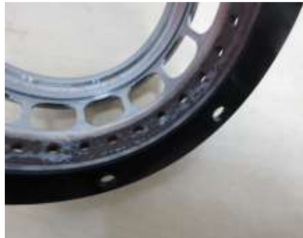
No.4 Brg: Corrosion on more than 30% of Area 1
