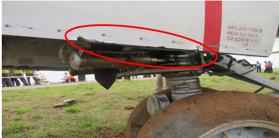
Pic 1: Damage on NLG left door
