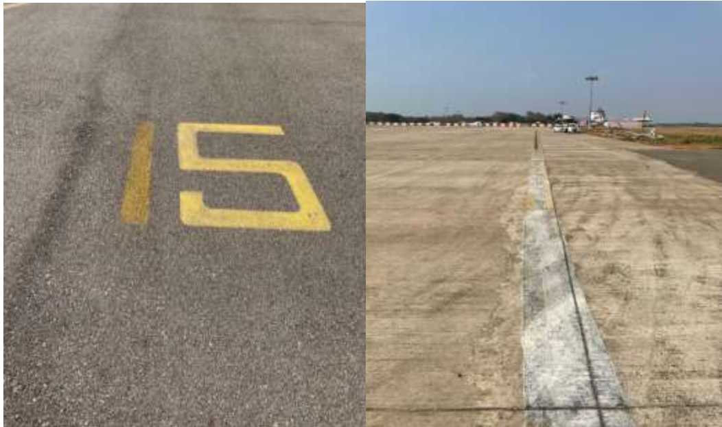
FIGURES: NON STANDARD MARKING AT AIRPORT (at the time of accident)
