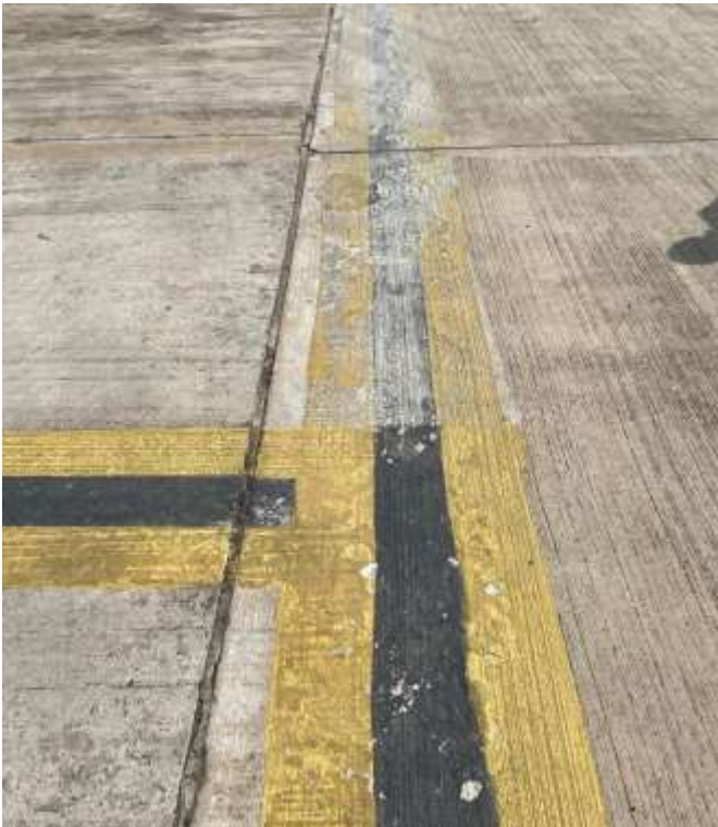
FIGURE: SHOWING SHOULDER EDGE MARKING AT VIJAYAWADA AIRPORT
