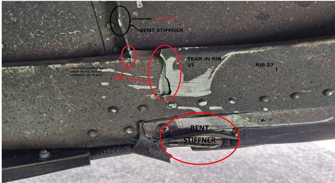
Figure2. Damage observed at LH landing gear bay structure.
